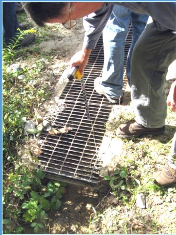
Homemade open-top box culvert (top)
